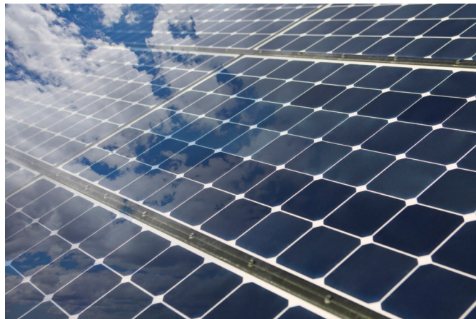
Figure 49: Large solar installations consist of hundreds of thousands of solar panels that must be arranged and wired.
